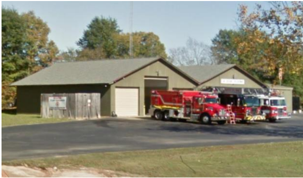
Figure 125: Flint-Gresham VFD, Station 1
